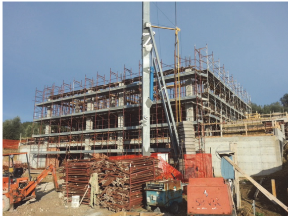
Fig. 2. Building under construction
